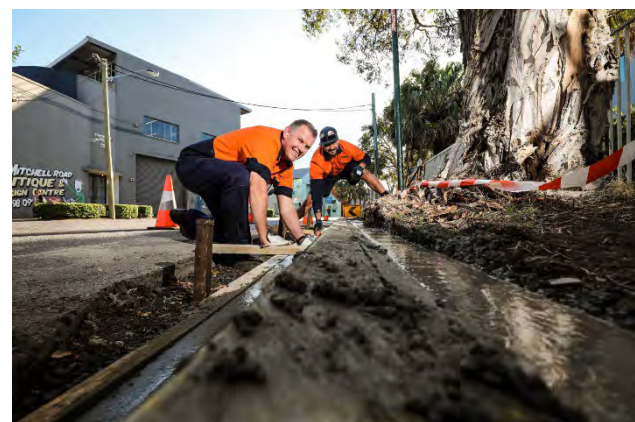
Image 26: Infrastructure Maintenance, Alexandria
