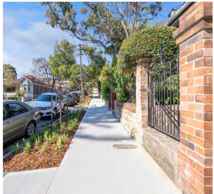
Images: Eglinton Road, Glebe Footway Renewal Works 2021
